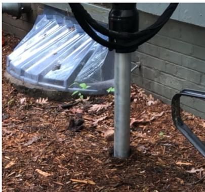
Should churning or augering occur without immediate correction, the screw should be removed and repositioned. If using the same hole is required, 3/8" "chip" gravel can be poured into the hole to re-establish the load-ability following the installation procedures described above. A maximum of 15 RPMs is advised and only with a mechanical driver capable of enough crowd to advance the screw as described above.
