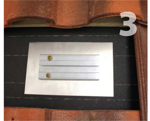
Install the base mount. Clean away dust and debris. (See instructions on pg 1)
