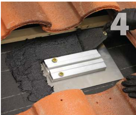
Apply 1/8" thick layer of roofing cement around the top and sides of the sub-flashing with at least 2" extending past the sides of the flashing onto the felt.
