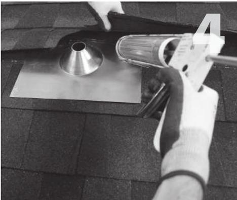
Slide flashing into place over drilled hole and apply a bead of sealant across the top side of the flashing under the 2nd shingle course. Be careful not to rip or tear shingles.
