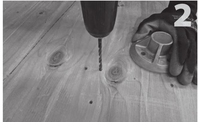
Drill both pilot holes with a 7/32-inch bit. Make sure to hold the drill square to the rafter. The lag bolts must be anchored into a structural member, so it is very important to hit the center of the rafter with your pilot holes. Fill the pilot holes with a sealant compatible with roofing materials.
