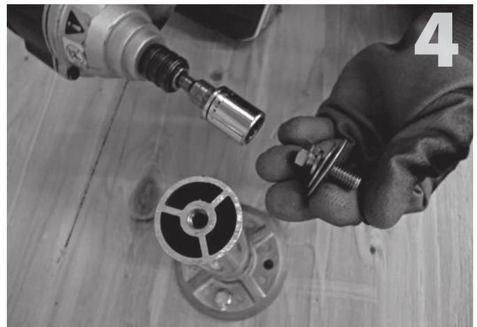
Attach the hardware (items 5-8) to the top of the post. (Be sure to seal off the post from weather exposure with the sealing washer (item 5), in the interim before racks are installed.) You are now ready to flash the mount, roof around it, and attach racking. Aluminum flashings for built-up roofs are available from Quick Mount PV in 4" and 8" cones (sold separately). For membrane roofs, be sure to use manufacturer-specified flashing and utilize the services of a certified roofer.
